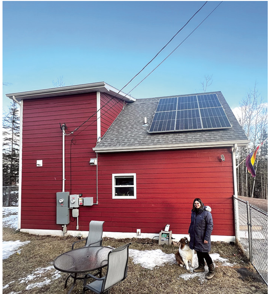
Sam with her pup in front of her home with new solar panels installed
