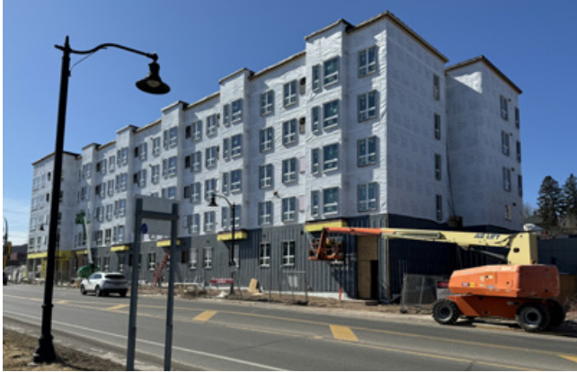
Brewery Creek Apartments, under construction
