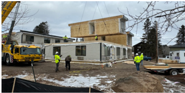
Modules being set for the Plover Place project
