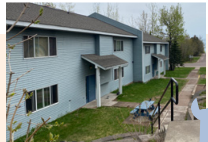
The Birchwood Apartment complex, beginning rehabilitation in 2024
