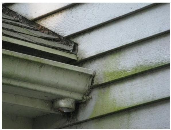
Lack of flashing can easily cause wall rotting and molding in walls
