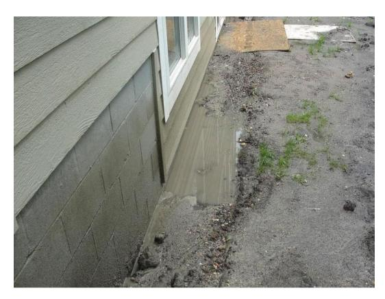
Standing water near the foundation is never a good sign and is an indication of a negative slope toward a home.
