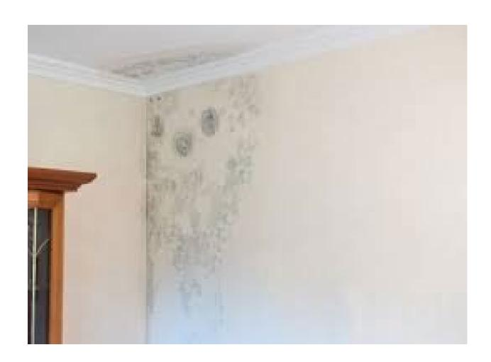
More than likely some roof valley damage that has run down the inside of the wall.
